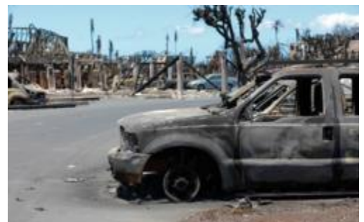
Damaged buildings and vehicles in Lahaina. [Spc. Sean Walker, photo.]
