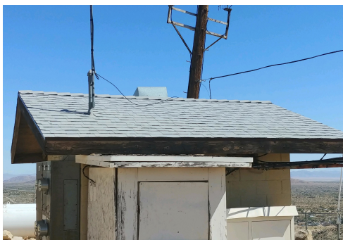
The new shingles installed. — Photo by N6GKB
