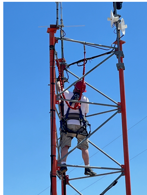
Chris WB6CDF repairs the repeater antenna's coax connection. — Photo by N6GKB
